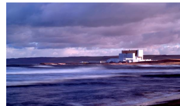
Torness Power Station
