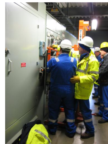
The Retrofit Operation at Torness
