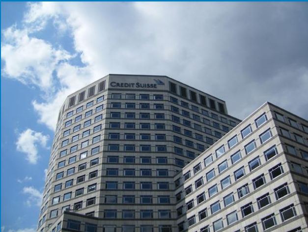
Credit Suisse, Canary Wharf
